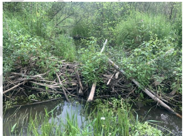
Photo 22: Beaver dam 125 m downstream of discharge location, breached, not a
