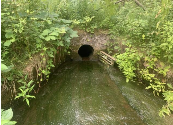
Photo 31: Looking at discharge structure
