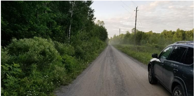
Photo 1: View south down access road leading to the Wastewater Treatment Plant.
